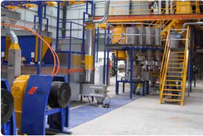
Big River Feeds SKIOLD 15tph pelleting complete plant Murray Bridge SA
