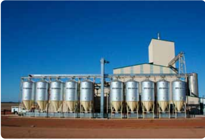
CEFN Feed SKIOLD 10tph pelleting complete plant Strathine QLD
